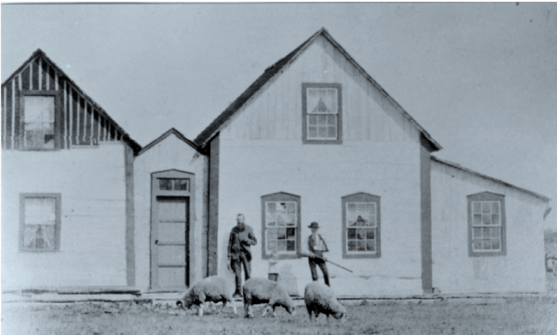
Figure 6 These gable-roofed log houses were joined, like their Icelandic predecessors with a narrow gabled entrance.
