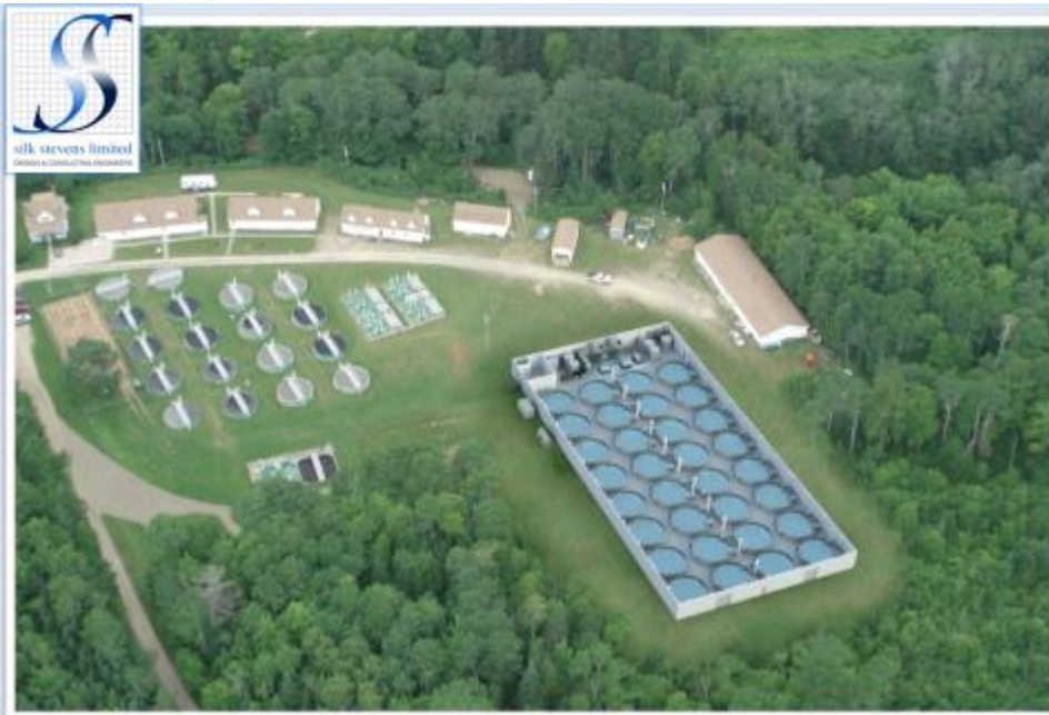
STURGEON AND SALMONID ENHANCEMENT FACILITY OPERATE AS FLOW THROUGH OR RECIRC - 7.5m TANKS
